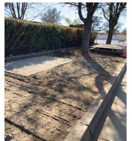
Madera Way Utility Relocation Construction (photo credit - Tasha Boutselis Camacho)
