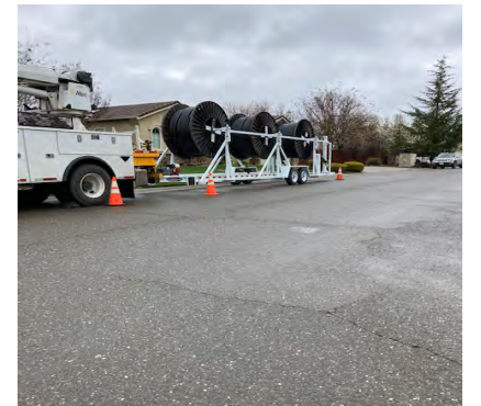
Summer Drive Utility Relocation Construction (photo credit - Tasha Boutselis Camacho)
