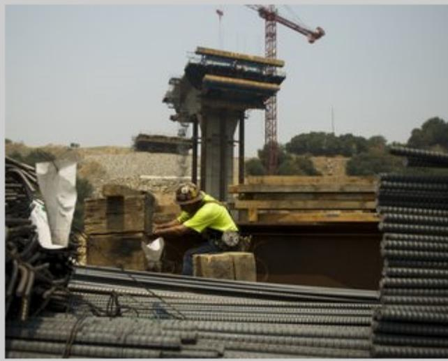
Mark Soulie, an ironworker on the Folsom Lake Crossing bridge project, ties together steel bars that will go in place as the center span is built.
